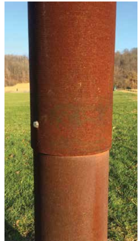
▶ Coated Finish Arc-applied zinc base coat with gray acrylic top coat
