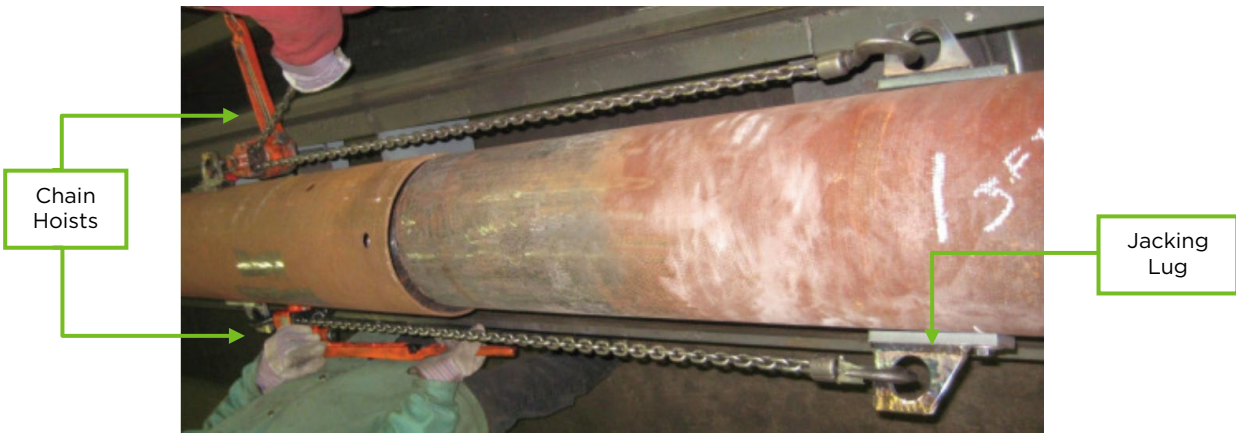
Figure 8: Chain Hoists Attached to Jacking Lugs
