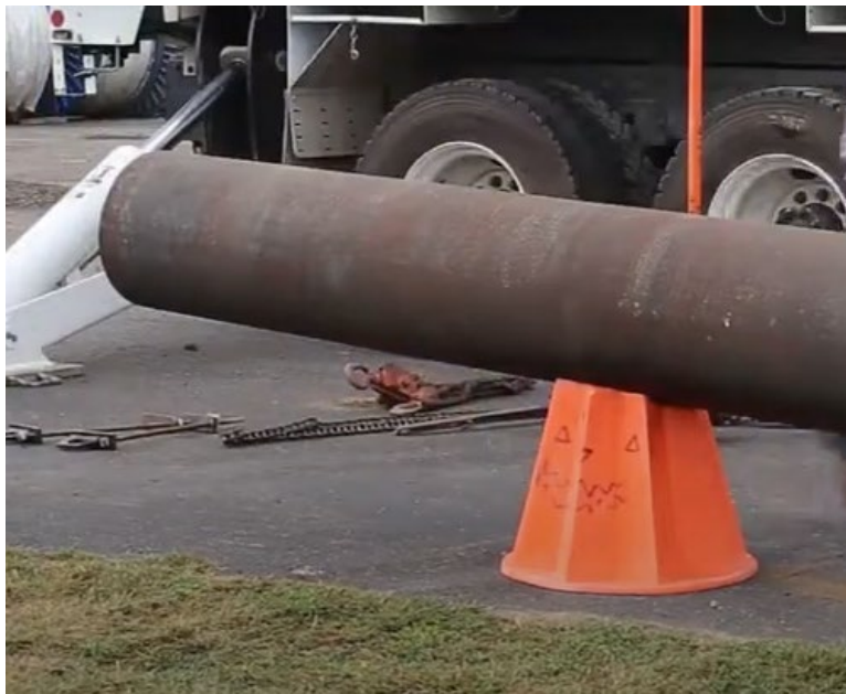
Figure 6: Inserting Section with Tip Elevated
