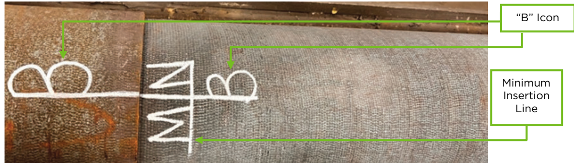
Figure 7: Quadrants Aligned at the Joint
